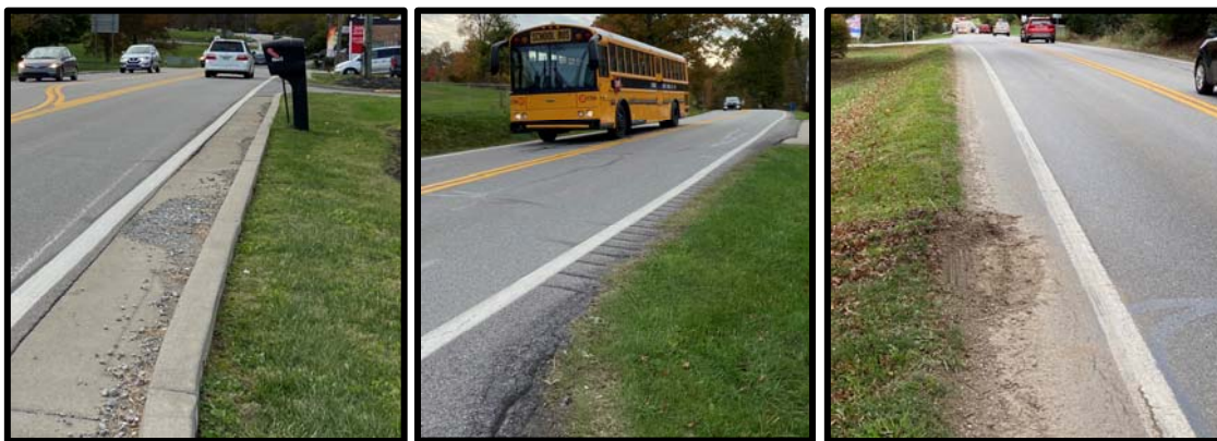
Figure 8. Representative Views of Shoulder Widths
