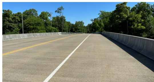
Figure 54: Clark Station Road Bridge
