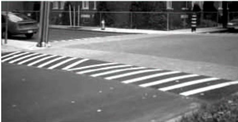
A raised intersection slows all vehicular movements through the intersection and improves pedestrian crossings in all directions.
