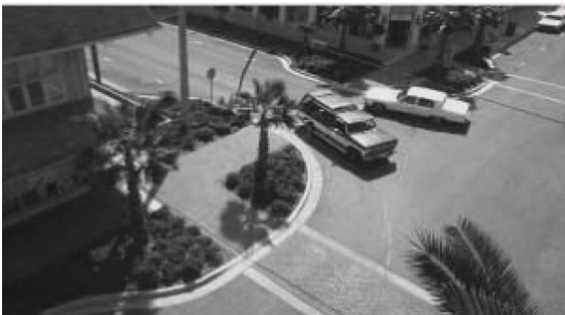
This curb extension in Venice, Florida, reduced motorist turning speeds by 6 to 8 miles/hour. Pedestrian crossing distance and time exposed to traffic was also reduced.
