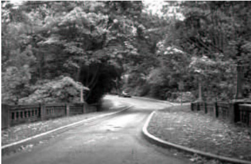
This choker on a two-way roadway in Seattle, Washington, narrows the street from two lanes to one. Traffic is forced to slow down and, in some cases, wait for an approaching vehicle to pass before proceeding.
