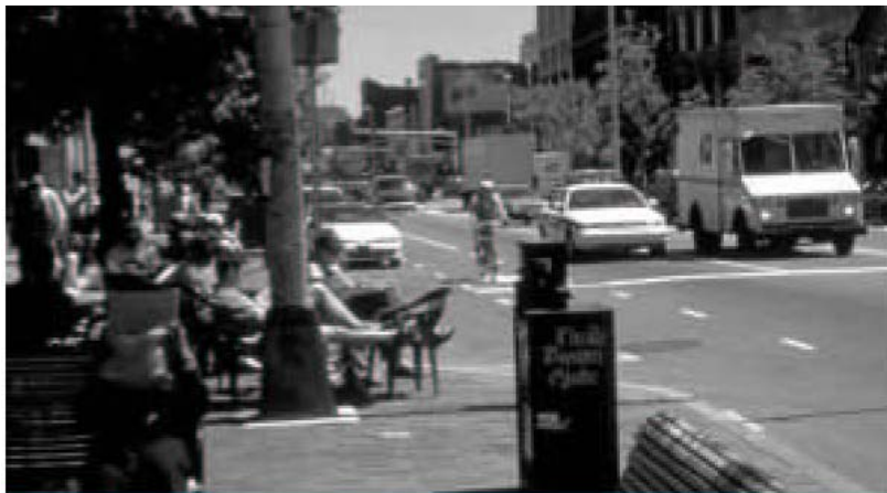
This street in Cambridge, Massachusetts was reduced from four lanes to three. The conversion introduced wider sidewalks, additional space for landscaping, street furniture and cafes, and bicycle lanes.
