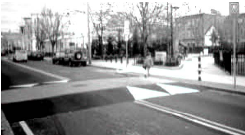
.A raised pedestrian crossing provides a continuous route for the pedestrian at the same level as the sidewalk. Pavement markings on the slope (inlay type) make the crossing visible to motorists.
