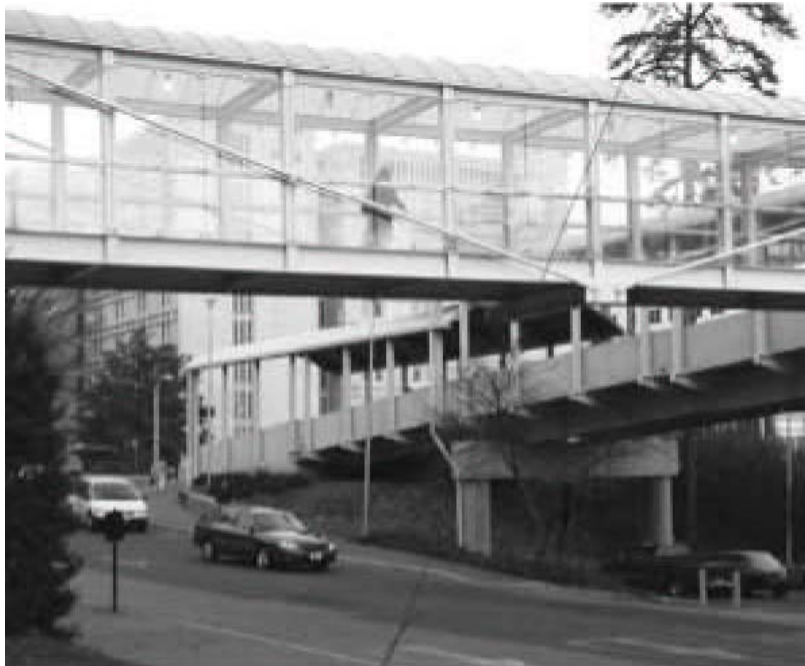
This pedestrian overpass takes advantage of existing topography and allows pedestrians to avoid conflicts with traffic at street level.
