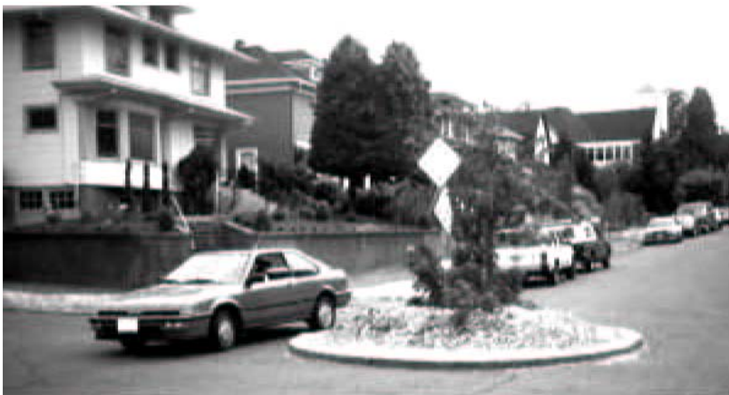
A traffic mini-circle helps reduce vehicle speeds, but still allows cars and emergency vehicles to pass through the intersection with little difficulty.
