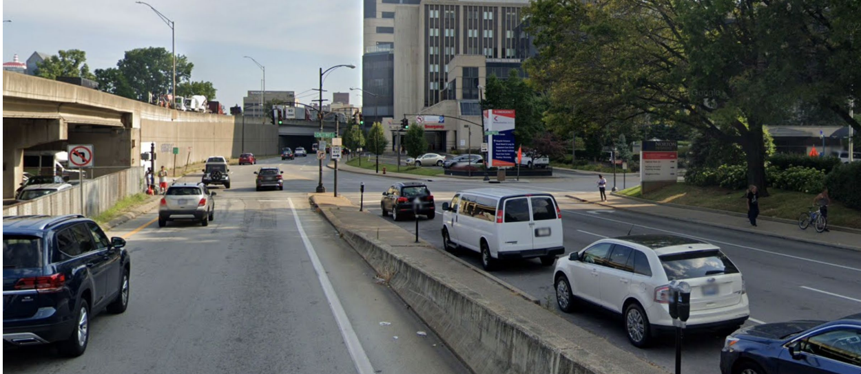
Figure 36: Brook Street Ramp (left) connection to Brook and Chestnut streets
