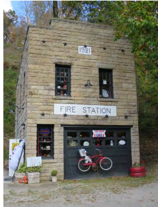
Historic fire station in Lynch, rehabilitated with the assistance of CDBG funding.
