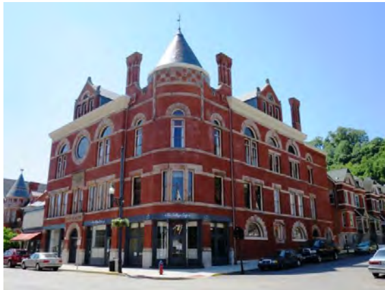
The Cox Building, Maysville, rehabilitated following a devastating fire in 2010.
