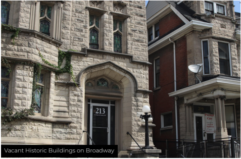
Vacant Historic Buildings on Broadway
