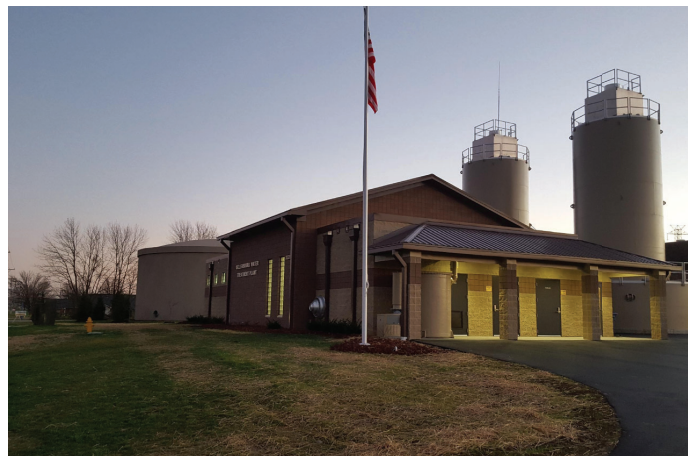
Sellersburg Water Plant Established November 2015
