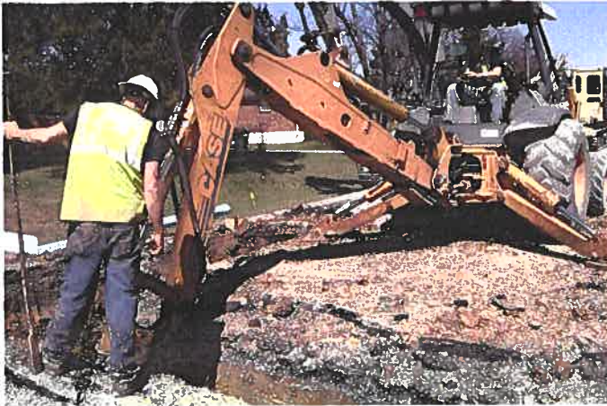
Recent Water Line Improvement Project
