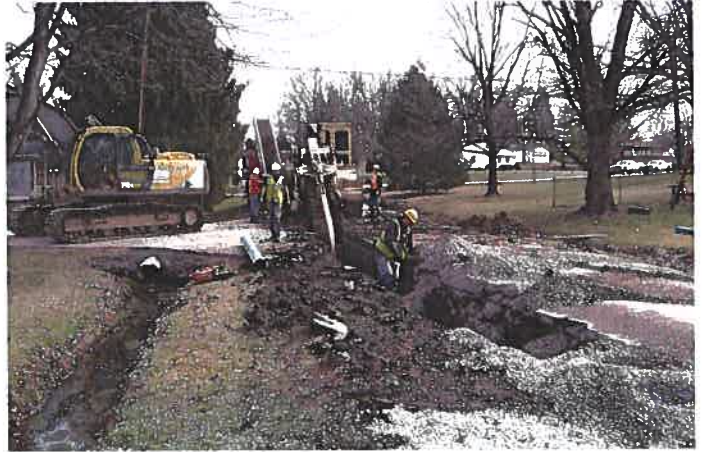
Recent Water Line Improvement Project
