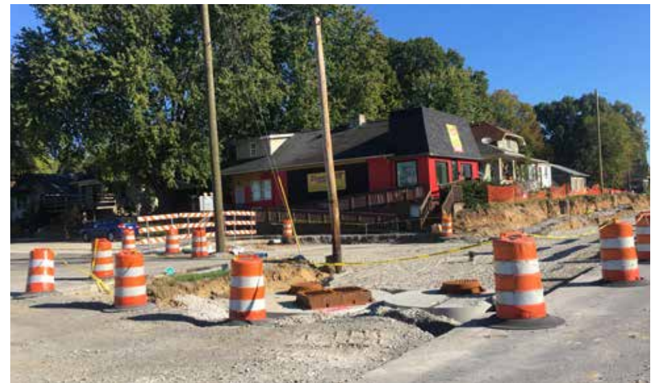
10TH STREET UNDER CONSTRUCTION
