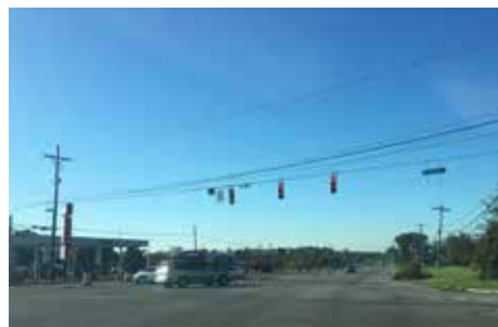
MISSING MULTI-MODAL INFRASTRUCTURE
