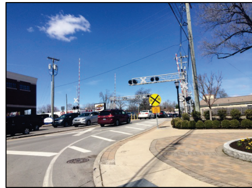
Figure 10: Railroad Crossing at Southern Terminus
