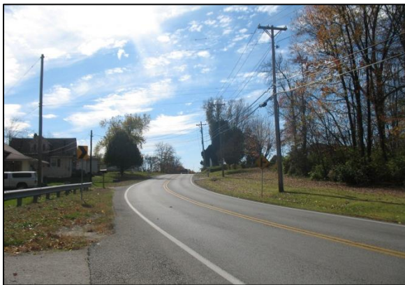
Manslick Road at Holly Park Drive looking to the south at one of several deficient vertical curves.
