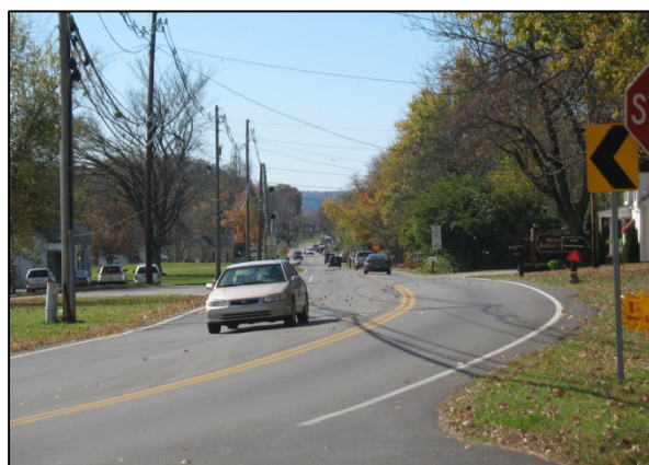
Narrow shoulders are present throughout the corridor.
