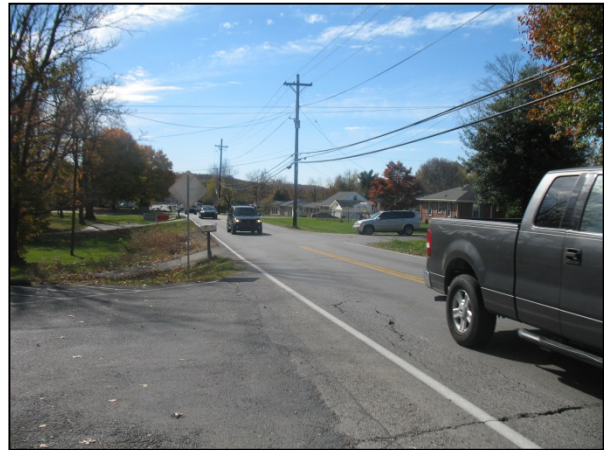
Densely-spaced driveways and side streets present safety concerns along KY 1931.
