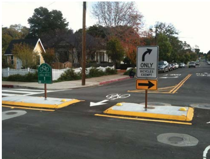
alternate forms of transportation. Using this feature will create safer neighborhoods by redirecting vehicular traffic to main thoroughfares and preventing cut-through scenarios.
