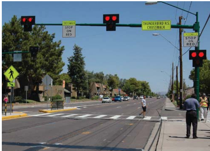
Utilize a hawk signal at busy roadway to provide extra protection for pedestrians crossing the road. These signals can be used at intersections or at mid-block.
