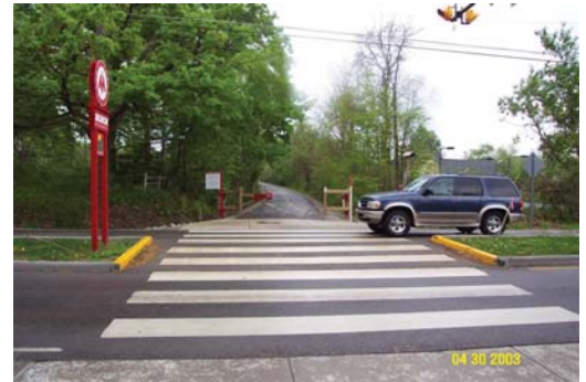
Example of a Street Crossing on the Monon Trail Carmel, Indiana
