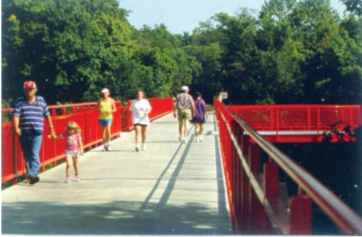
Example of a Standard Bridge on the Monon Trail Indianapolis, Indiana
