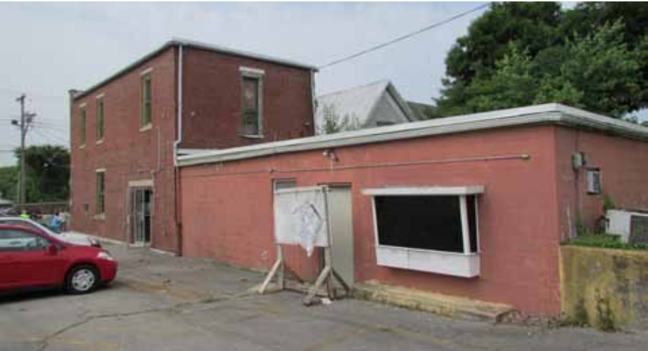
Context Photo - view of east elevation
