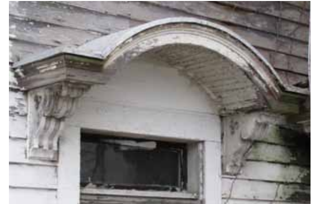
Arched hood over entry door
