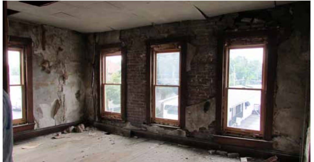
Bank building interior view
