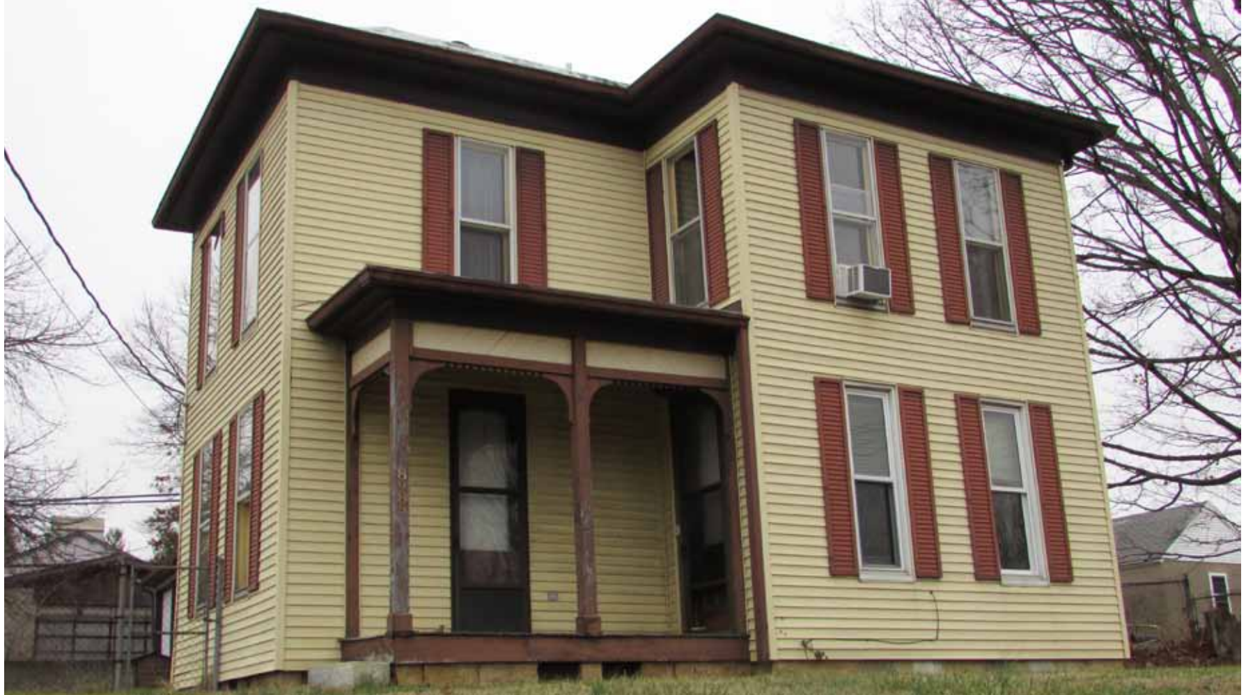
Note the overhanging eaves and detailed brackets at the porch
