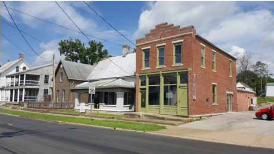
Context Photo - view looking northwest
