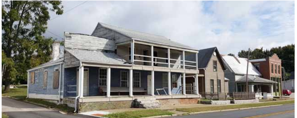
Wolfe Hotel with classic Greek Revival features – original porch columns now lost
