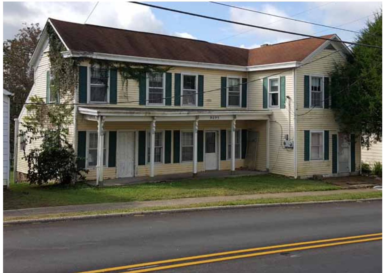
9093 State Road 64 - Note the characteristic Greek Revival cornice returns and wide cornice boards
