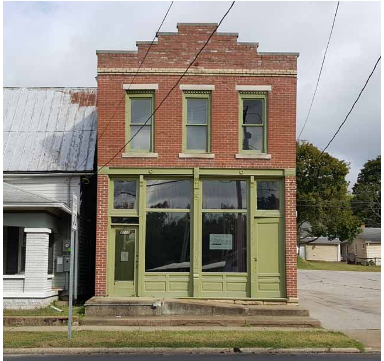
9110 State Road 64 - Georgetown Bank
