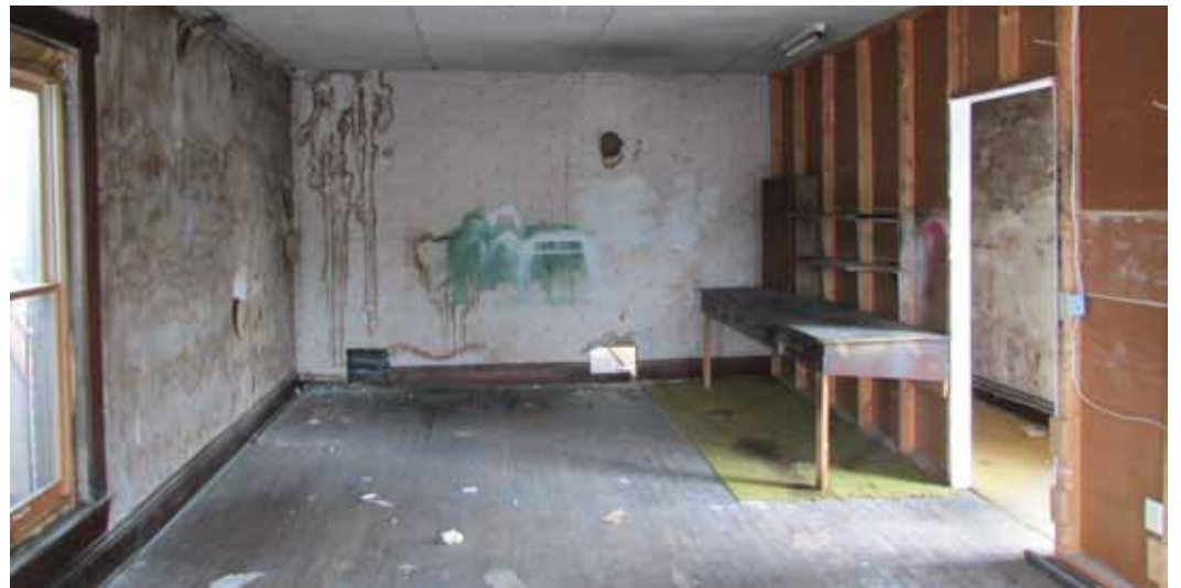
Bank building interior view
