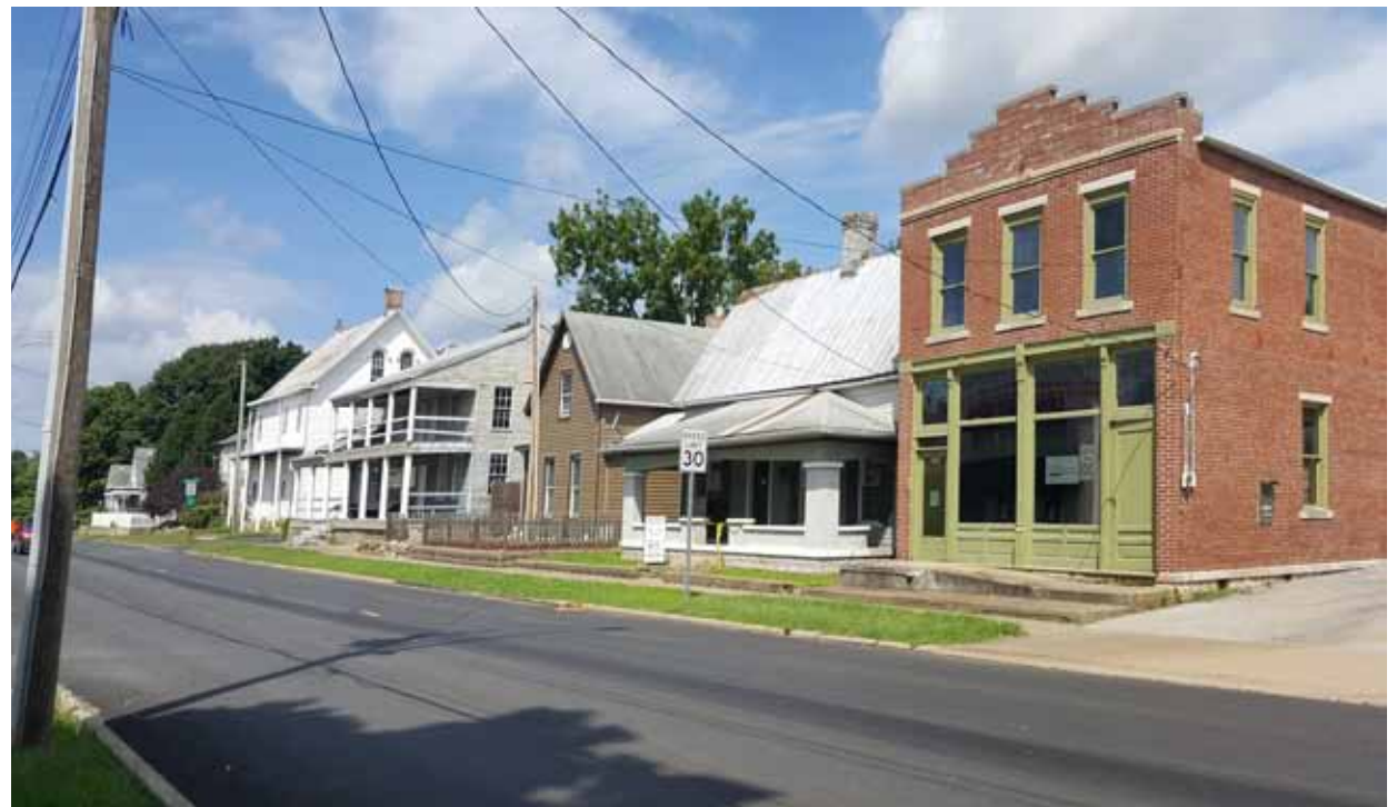
Views looking west along State Road 64/Main Street
