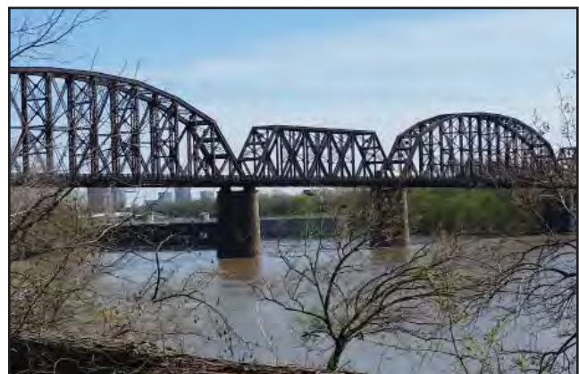
K&I Railroad Bridge
