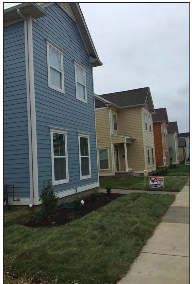
New home construction in the midtown area of New Albany
