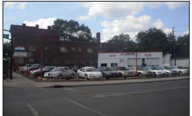
A used car lot in an urban environment is an example of a use that may not be desirable in a community and could be discouraged with form-based ordinances
