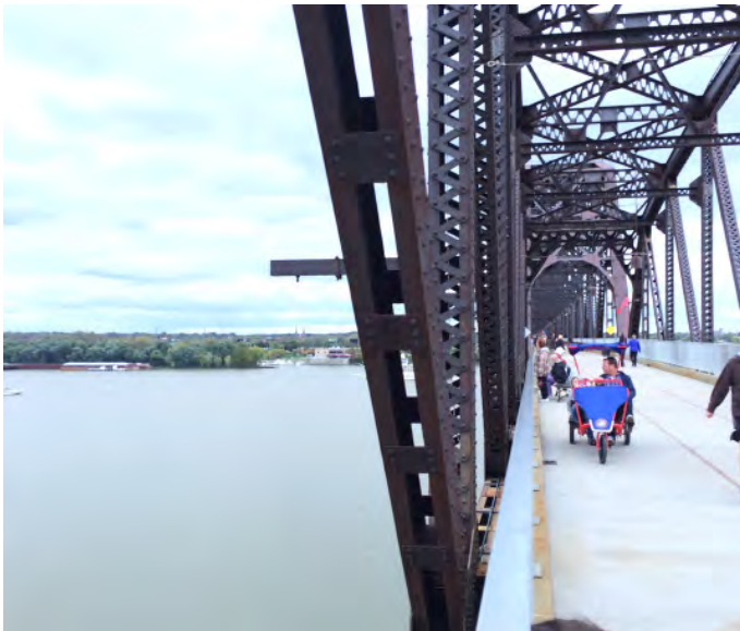
Big Four Pedestrian Bridge
