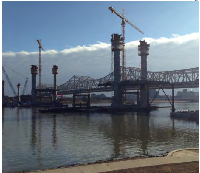
Construction of Downtown Crossing
