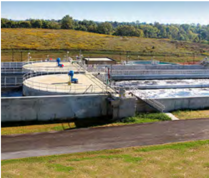
Jeffersonville Wastewater Treatment Plant
