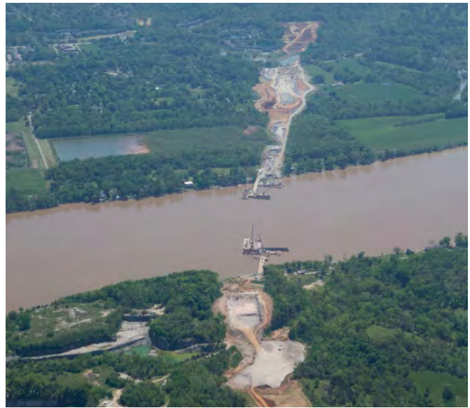
Road Construction for new East End Crossing
