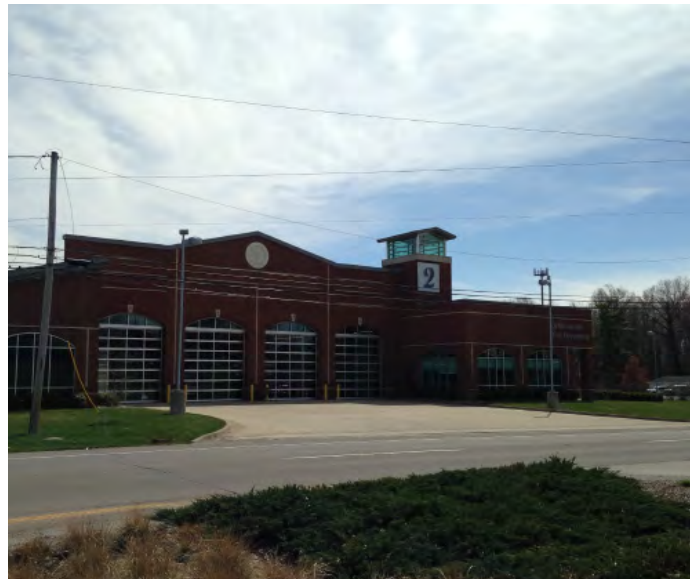
Jeffersonville Fire Station
