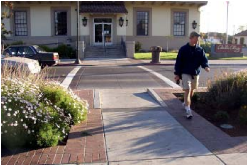
Sidewalk with ADA accessible ramp
