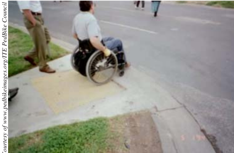
An ADA accessible curb ramp
