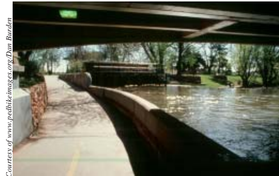
Multi-use underpass alongside a creek.
