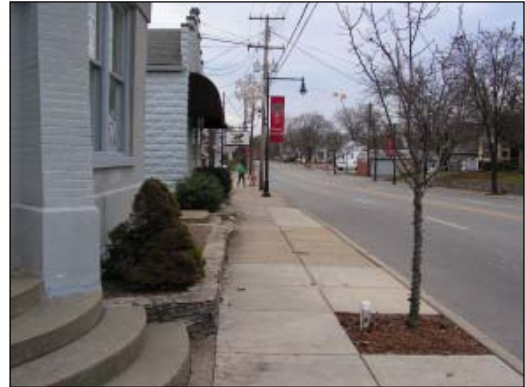
Existing Sidewalk - Watterson Trail
