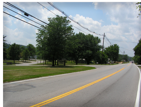
Figure 21: St. Andrews Church Road looking west at Trunnell Elementary School
