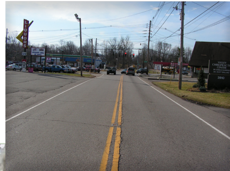
Figure 11: East Pages Lane looking south to the 3rd Street Road Intersection
