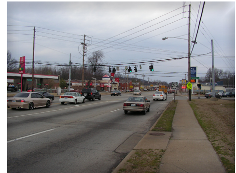
Figure 16: New Cut looking north to the 3rd Street Road intersection
