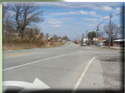
Picture 8: 3rd Street Road looking northeast at the Manslick Road intersection
