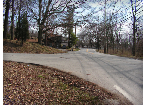
Figure 3: 3rd Street Road looking east at James Hill Curve Intersection
