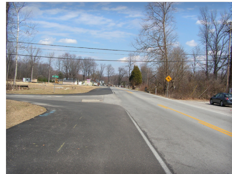
Figure 39: 3rd Street Road looking northbound at McNair Road Intersection
