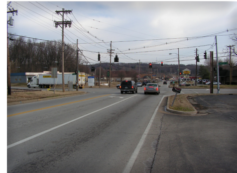
Figure 34: 3rd Street Road looking north to Stonestreet intersection
