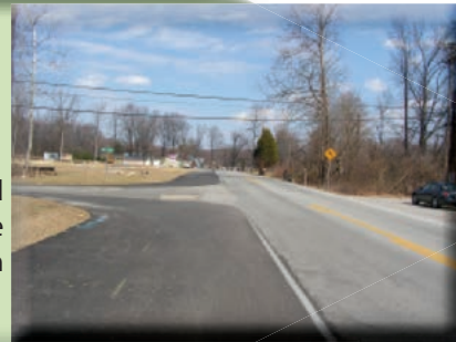
Picture 14: 3rd Street Road looking northeast at the McNair intersection
