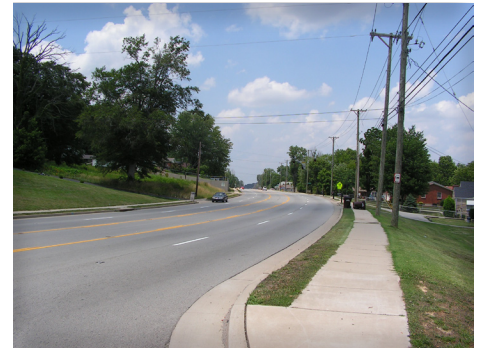
Figure 22: New Cut Road corridor looking north
