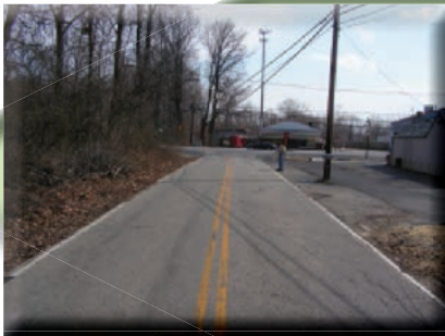
Picture 13: McNair Road looking southeast to the 3rd Street Road intersection
