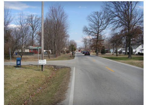
Figure 45: 3rd Street Road looking north
