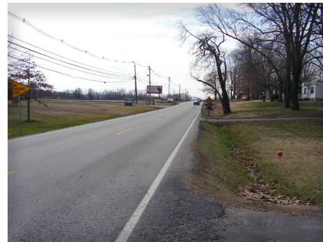
Figure 15: 3rd Street Road looking south from Wisertown Road
