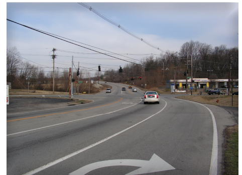
Figure 35: Stonestreet looking west at 3rd Street Road intersection
