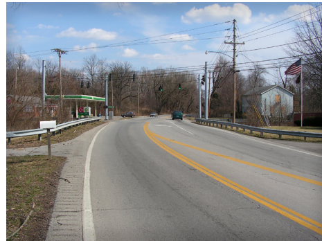
Figure 18: 3rd Street Road looking northbound to the Arnoldtown Road Intersection
