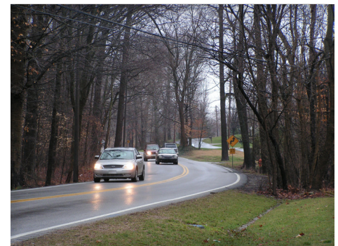
Figure 50: Palatka Road looking east from Iroquois Park Road
