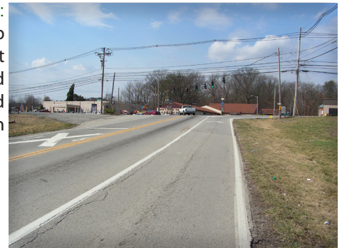
Figure 38: Outer Loop looking west at the 3rd Street Road intersection
