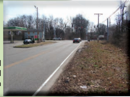
Picture 6: Arnoldtown Road looking southeast to the 3rd Street Road intersection
