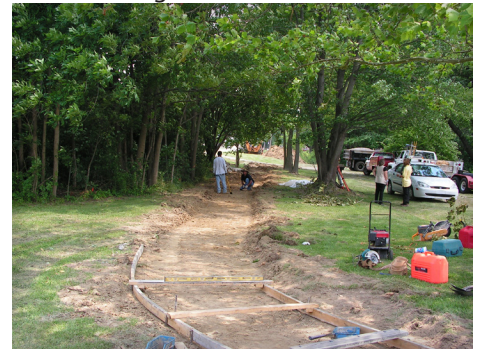
Figure 48: Sidewalk under construction near Doss High School
