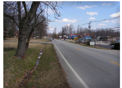
Figure 46: 3rd Street Road looking north from Wisertown Road intersection
