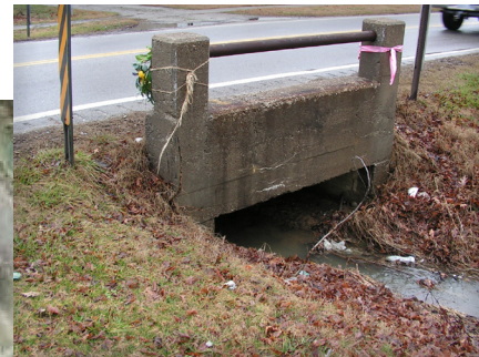
Figure 6: The headwall on the east side of Southside Drive
