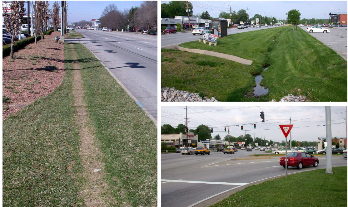
Figure 5: Shelbyville Rd is a popular commercial corridor, yet it lacks many basic pedestrian accommodations. Few sidewalks are present, forcing pedestrians to beat their own path (right). A bus stop provides no connection to nearby shopping centers (far upper right). Multiple free-flowing travel lanes make crossing this side street difficult (far lower right).
