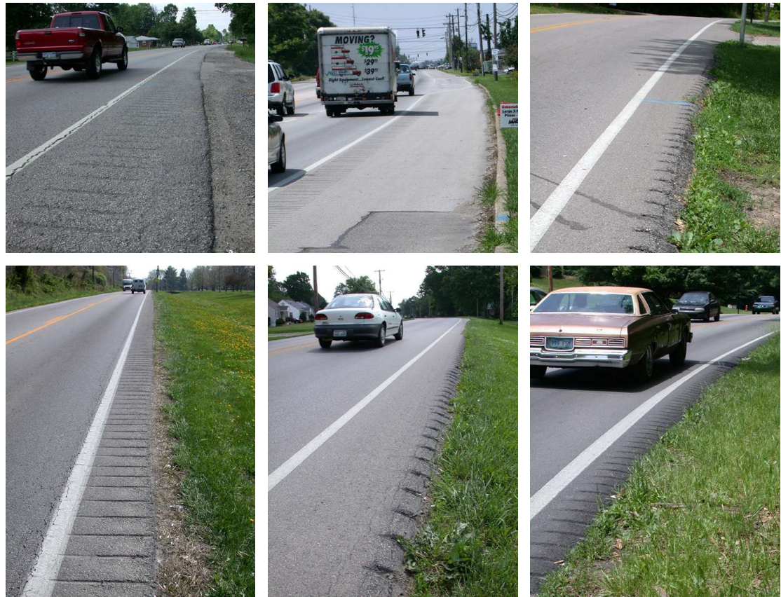
Figure 7: Shoulder rumble strips are found throughout Louisville Metro. On some wide paved shoulders, there is enough space to accommodate bicyclists despite the presence of rumble strips (upper middle); however, in many cases rumble strips are not bicycle friendly (upper and lower right). In other cases, rumble strips are applied to narrow shoulders or to the extreme edge of the shoulder, providing little, if any, useful warning for motorists deviating from their lane (lower middle, upper and lower far right).
