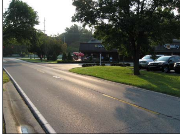
Looking at the driveway into Prospect Point (and Java Brewing Company) from Sedgewicke Drive at the River Road intersection.
