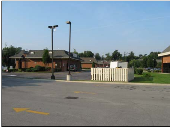
From behind Circle K, looking at the site of vehicular connection to the Water Works Car Wash lot.
