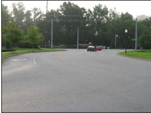
Looking south at the Timber Ridge Drive and US 42 intersection.
