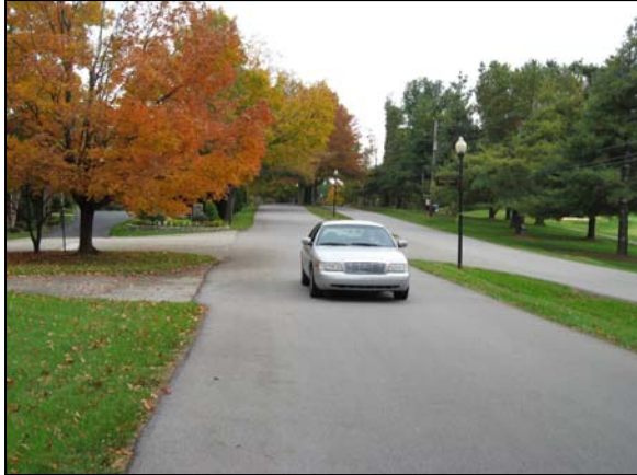
Hunting Creek Drive showing the width and lack of striping.
