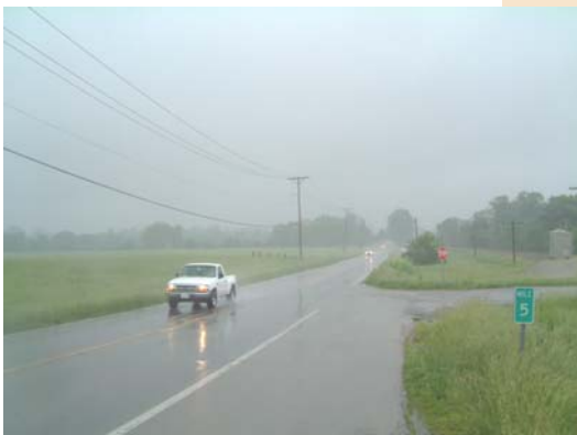
Looking East along KY 146 between KY 329 and KY 393
