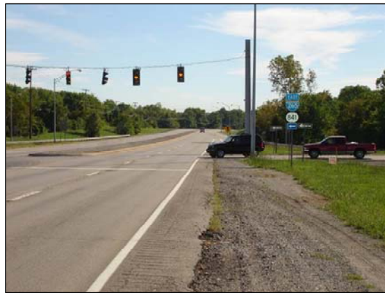
Southbound Gene Snyder Freeway Off-Ramp to Taylorsville Road
