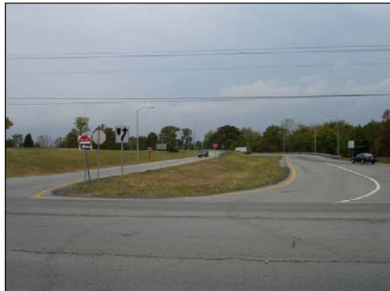
I-71 Southbound Ramps
