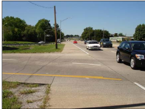
Northbound Taylorsville Road On-Ramp to Watterson Expressway Westbound (looking north)
