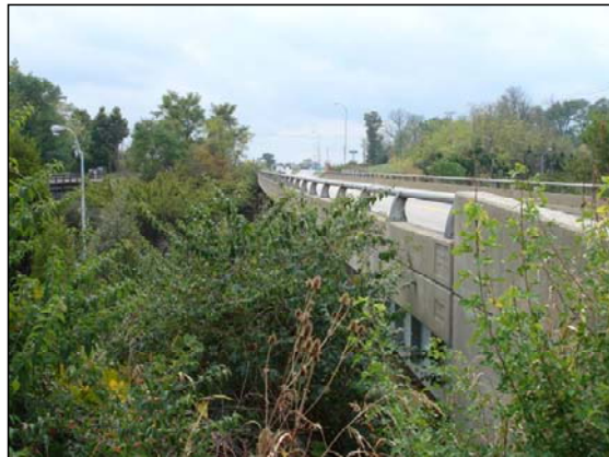
KY 146 Bridge Over I-71
