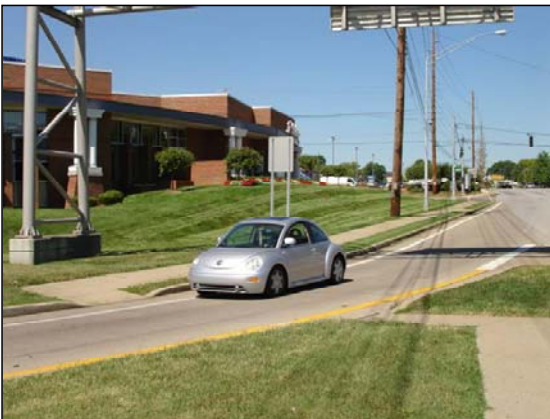
Southbound Bardstown Road On-Ramp to Westbound Watterson Expressway
