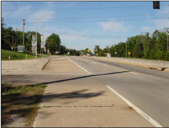
Taylorsville Road On-Ramp to Southbound Gene Snyder Freeway
