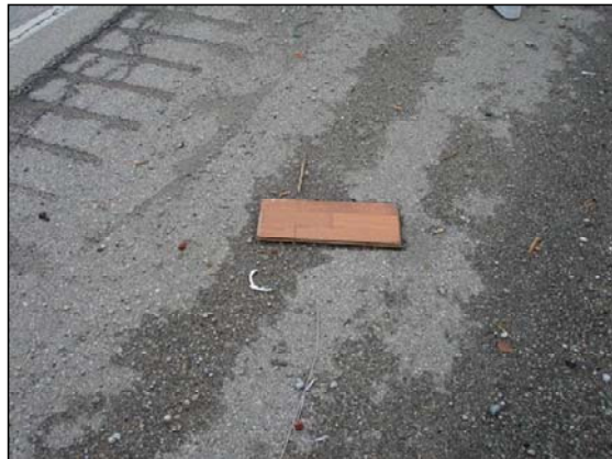
Trash Obstacle in Shoulder
