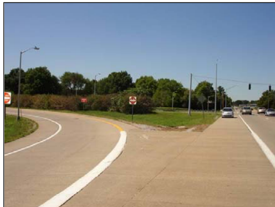
Westbound Watterson Expressway Off-Ramp to Southbound Taylorsville Road
