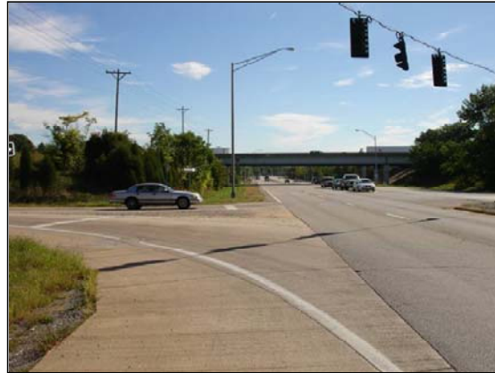
Southbound Gene Snyder Freeway Off-Ramp to Taylorsville Road
