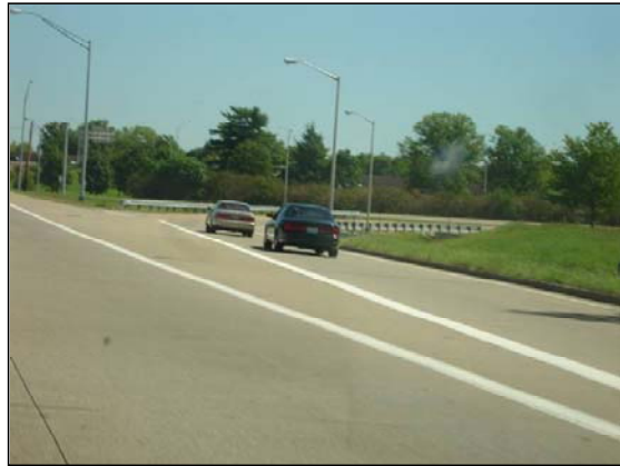
Southbound Taylorsville Road On-Ramp to Eastbound Watterson Expressway
