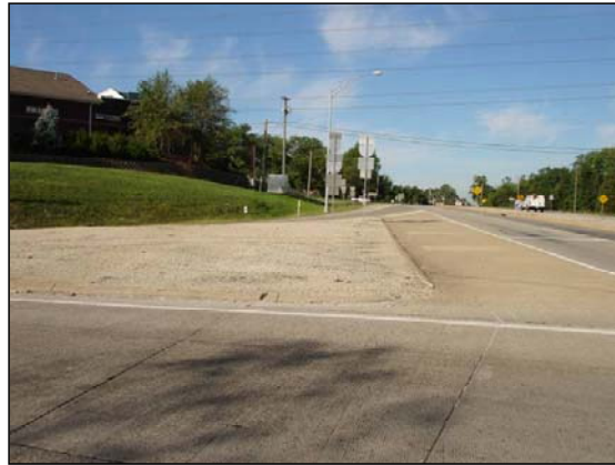
Taylorsville Road On-Ramp to Southbound Gene Snyder Freeway
