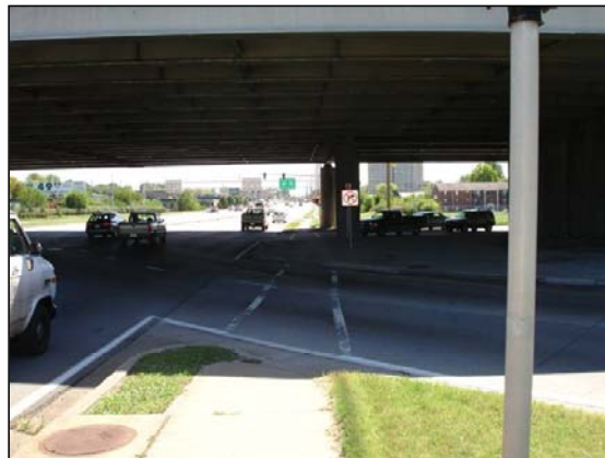
Northbound Bardstown Road On-Ramp to Westbound Watterson Expressway – Crosswalk
