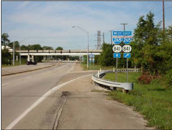
Westbound Taylorsville Road On-Ramp to Northbound Gene Snyder Freeway
