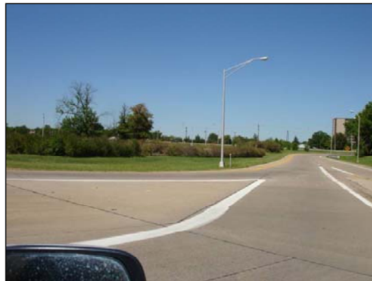
Triple Entry Taylorsville Road On-Ramp to Eastbound Watterson Expressway
