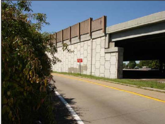
Eastbound Watterson Expressway Off-Ramp to Southbound Taylorsville Road
