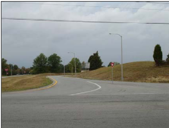
I-71 Northbound On-Ramp and KY 146
