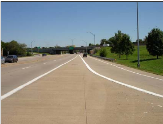
Westbound Watterson Expressway Off-Ramp to Southbound Taylorsville Road
