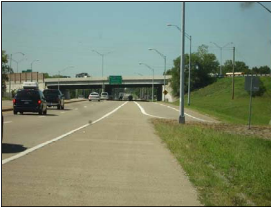
Northbound Taylorsville Road Off-Ramp to Westbound Watterson Expressway (looking south)
