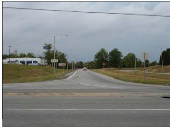
I-71 Northbound Off-Ramp to KY 146
