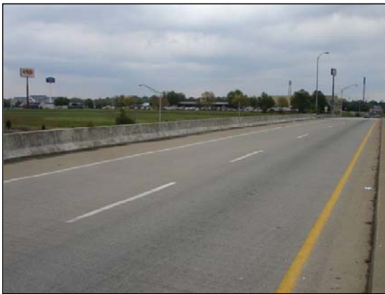
KY 1526 Bridge over I-65
