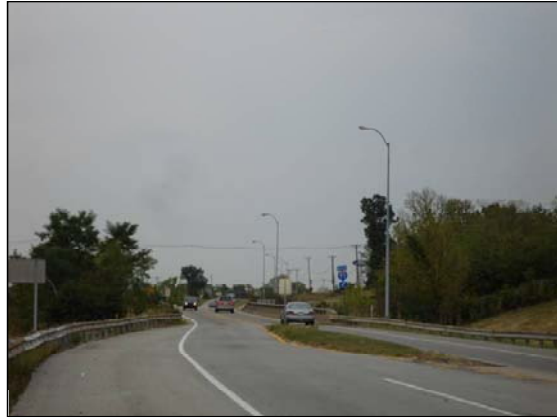
KY 146 Approaching the Bridge Over I-71
