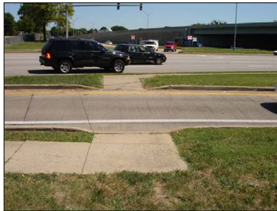
Southbound Bardstown Road On-Ramp to Westbound Watterson Expressway - 90 degree sidewalk
