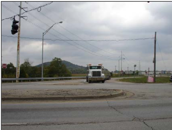
Southbound I-65 Off-Ramp to KY 1526
