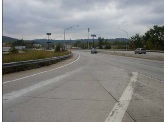
KY 1526 On-Ramp to Southbound I-65
