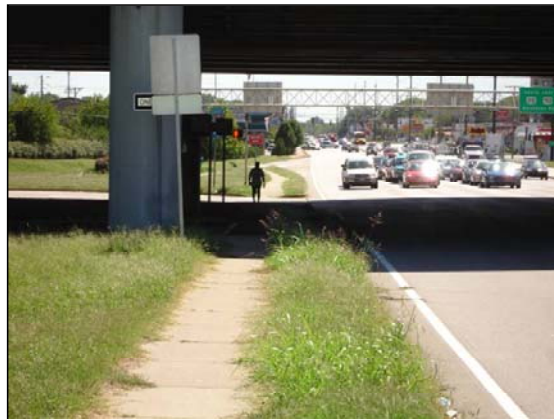
Westbound Watterson Expressway Off-Ramp to Southbound Bardstown Road
