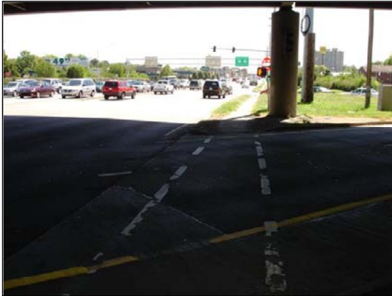
Eastbound Watterson Expressway Off-Ramp to Northbound Bardstown Road
