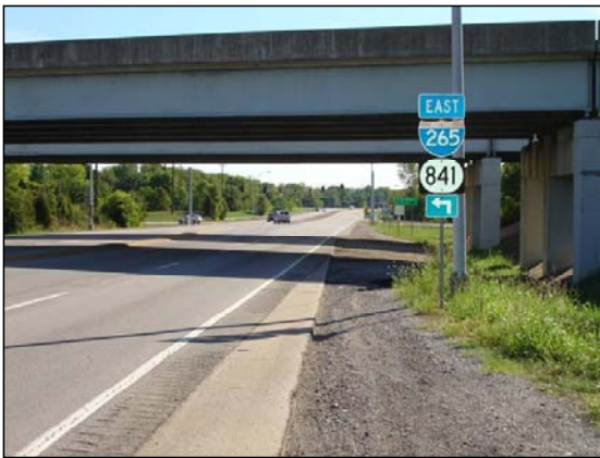
Eastbound Taylorsville Road
