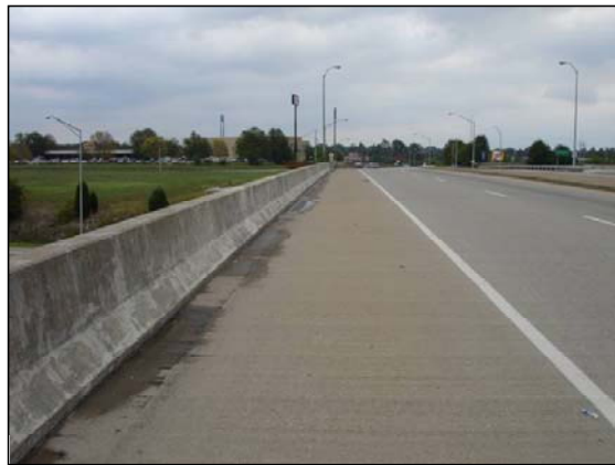
Shoulder of KY 1526 Bridge over I-65
