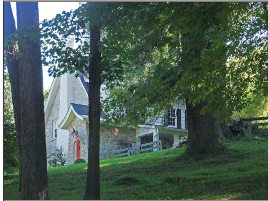
Figure 22. East-northeasterly view of James T. Taylor/James W. Chandler House (JF 784).
