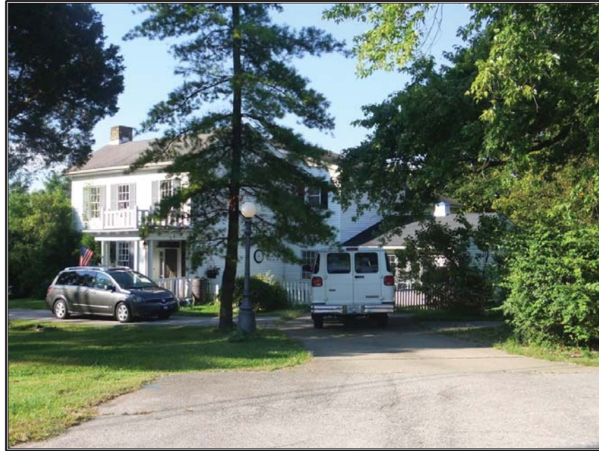
Figure 25. Southwesterly view of potentially eligible house at 4000 Hopewell Road (JF 204).
