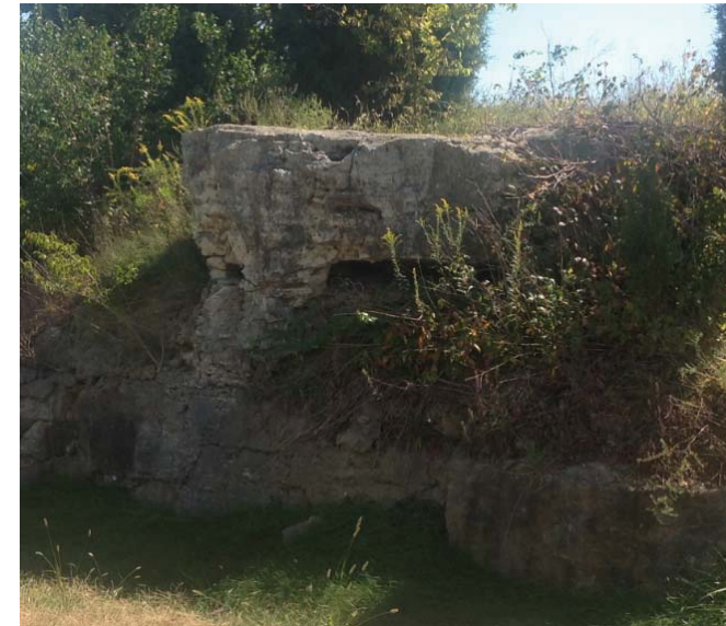
Example of Karst in Louisville Limestone in Rock Cut
