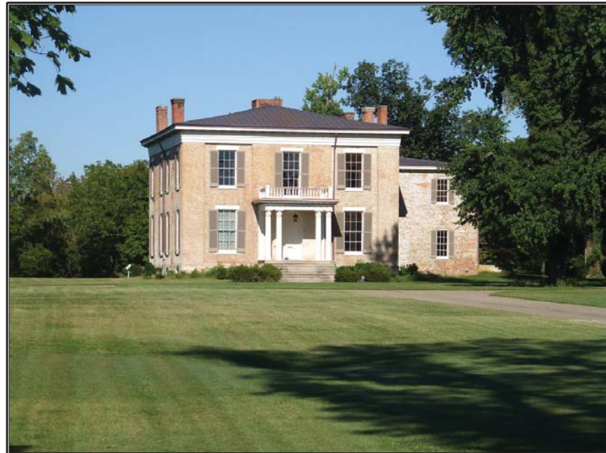
Figure 16. Northwesterly view of Rosewell (JF 452).
