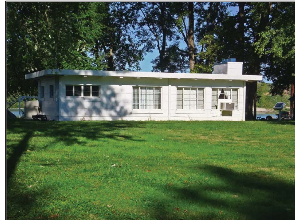
Figure 21. North-northwesterly view of John Determann House (JF 843).
