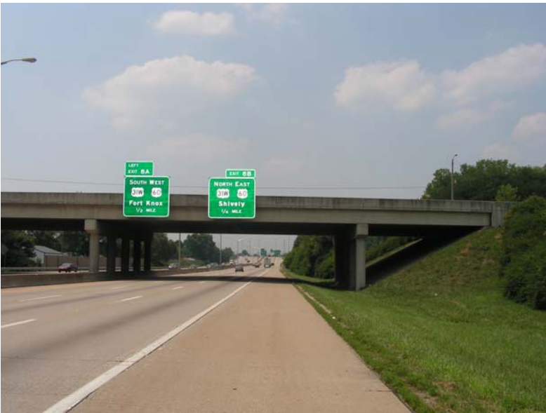
Photo 14 I-264 looking west at Manslick Rd Bridge
