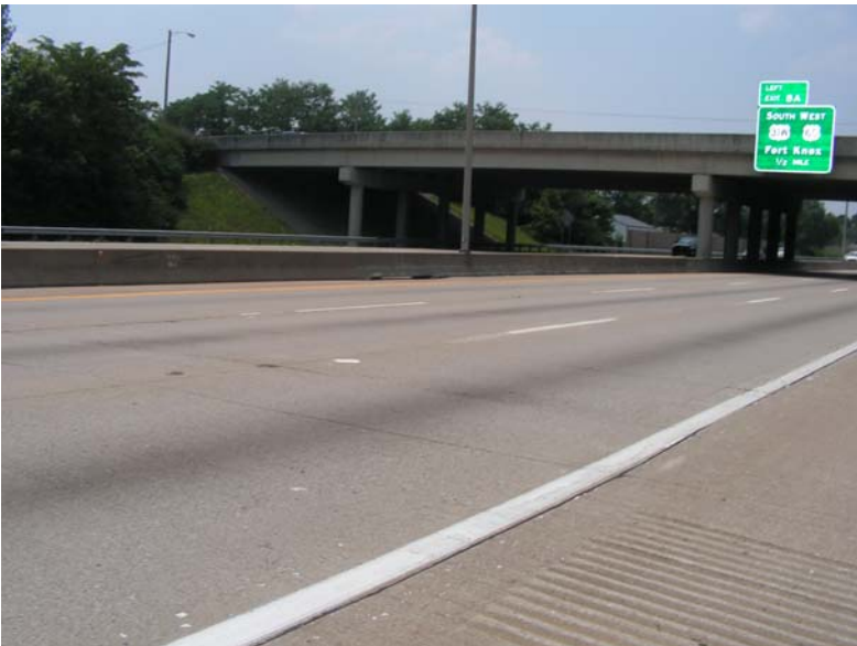
Photo 15 I-264 looking west at Manslick Rd Bridge
