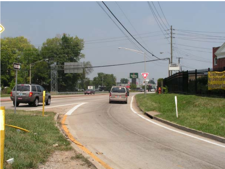
Photo 24 End of I-264 ramp to NB Dixie
