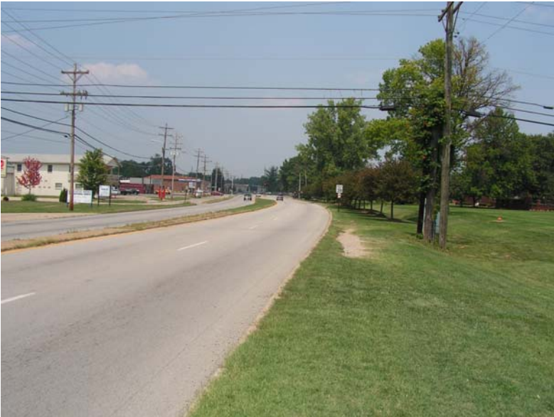
Photo 32 Manslick Road looking north, north of I-264
