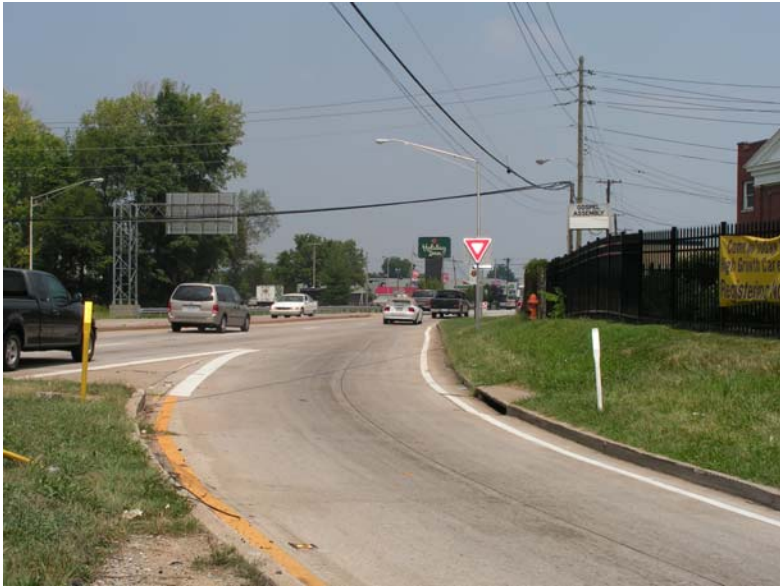
Photo 25 End of I-264 ramp to NB Dixie
