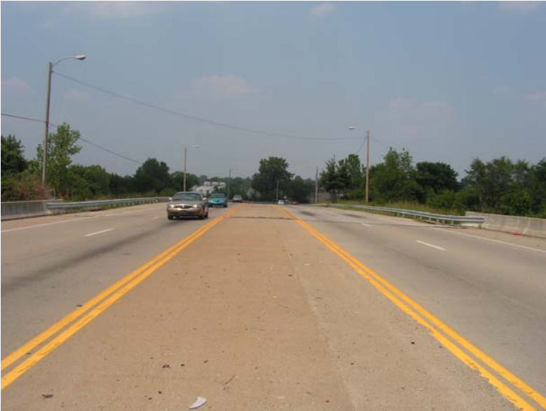
Photo 33 Manslick Road bridge over I-264, looking north
