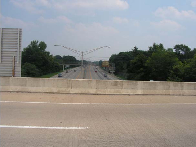
Photo 31 Manslick Road Bridge and I-264 looking east
