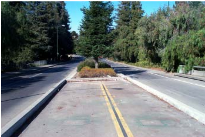
A roadway on a diet; recently narrowed from four to two-lanes.
