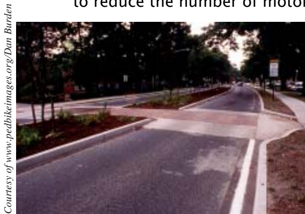
Example of an elevated cross walk/speed table with a pedestrian refuge area.
