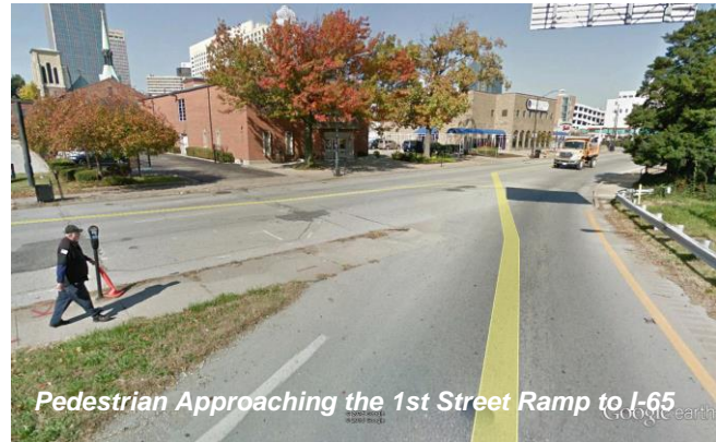
Figure 3.4-21: 1 st Street Ramp
