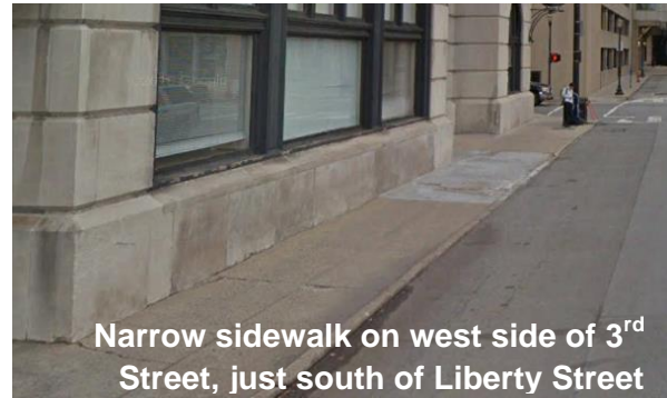
Figure 3.1-2: Third Street Sidewalk
