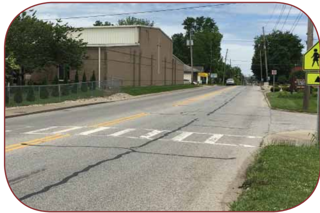
US 31 through Sellersburg near St. Paul Street Credit: HWC Engineering
