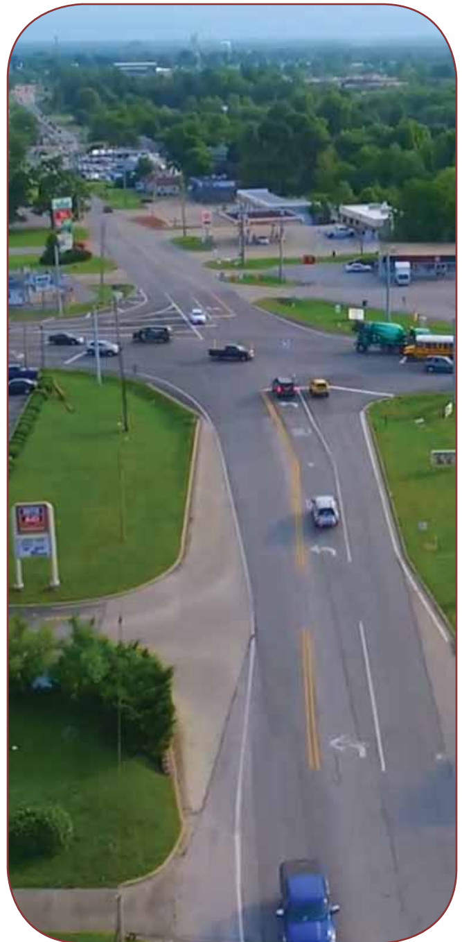
CR 311 at SR 60 Credit: HWC Engineering
