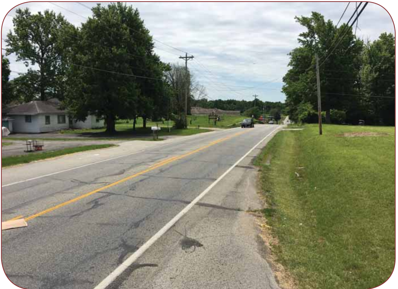
CR 311 north of County Line Road Credit: HWC Engineering
