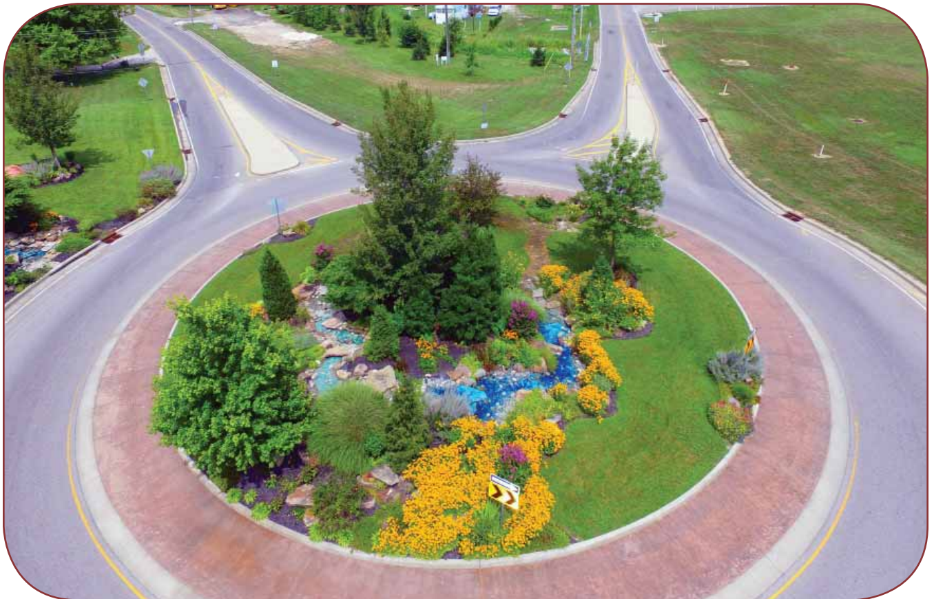
A roundabout at CR 403 provides an opportunity for a signature gateway into Sellersburg, while also greatly reducing congestion and efficiency through the intersection. While the roundabout above in Princeton, IN is only a single lane roundabout, it highlights how a water feature and landscaping can serve as a gateway into the community Credit: HWC Engineering.
