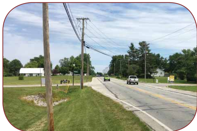
CR 311 at Westmont Drive Credit: HWC Engineering
