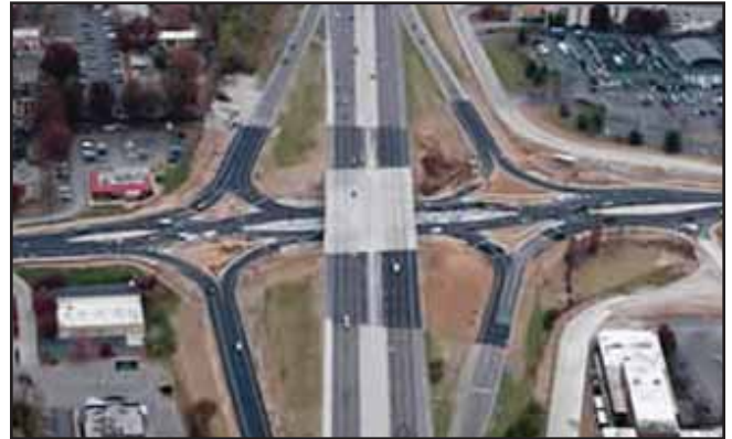
Diverging diamond interchange Credit: www.modot.org
