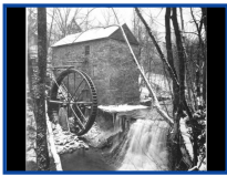
Wolf Pen Branch Mill (pictured) is located at 5824 Chamberlain Lane.
